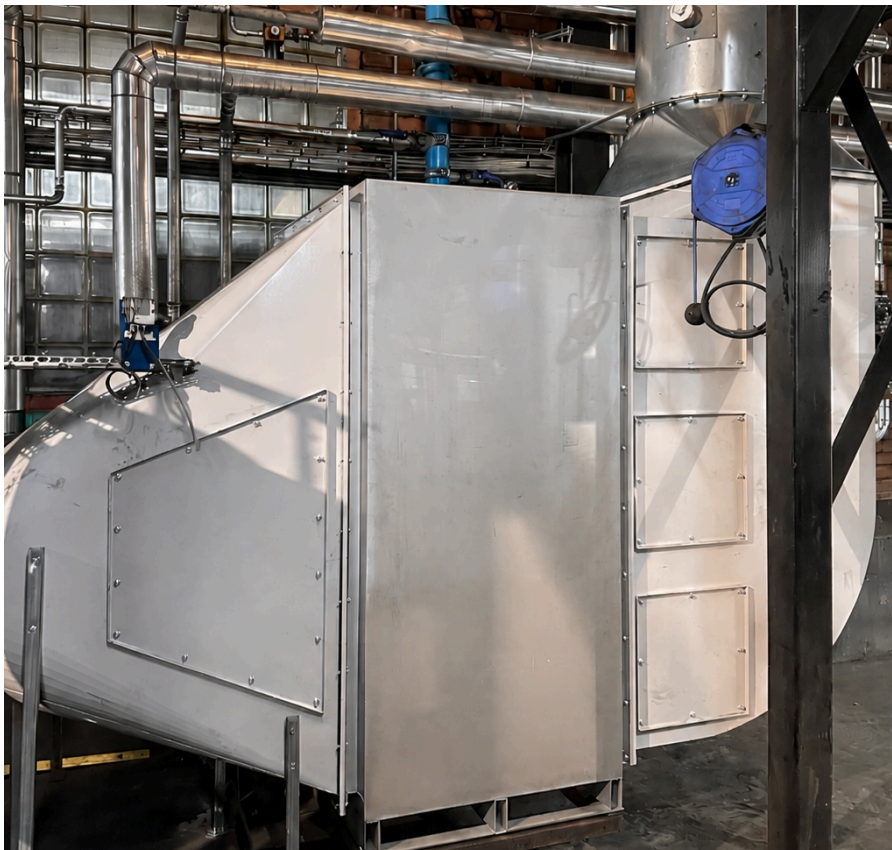
Lepido technology installed on-site in Bruzaholms sand cooler exhaust.
